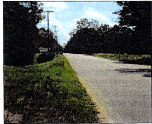
Site Visit: Paved Road
